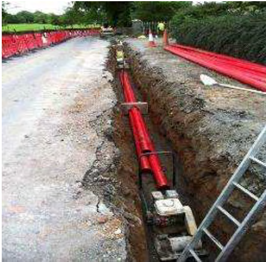
Image 2-1: Example of 110kV Underground Duct Installation
